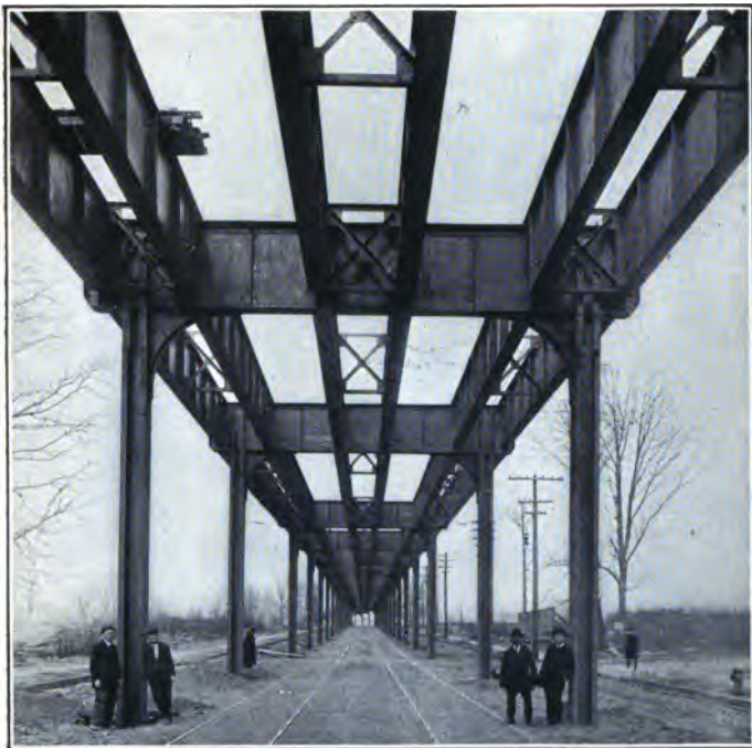
ELEVATED RAILROAD, STEEL STRUCTURE
